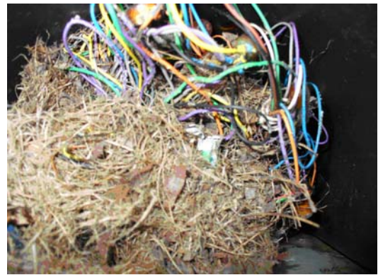
Photo 18: Mouse nest in 1970's junction box closest to lightning strike.
