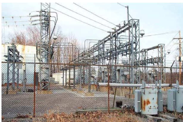
Photo 4. Sawmill Run Preparation Plant Substation
