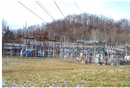
Photo 3. French Creek Substation
