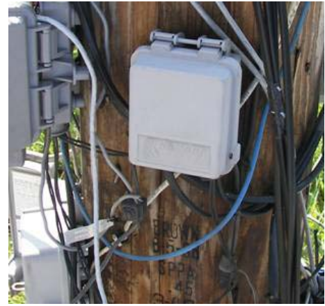
Photo 22: Ground Connection On Pole For Distribution Box
