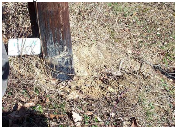
Photo 11. Disturbance at base of pole with the damaged insulators
