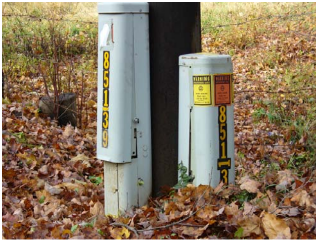
Photo 16: Junction boxes of the 1970's buried line and the 1981 buried line.
