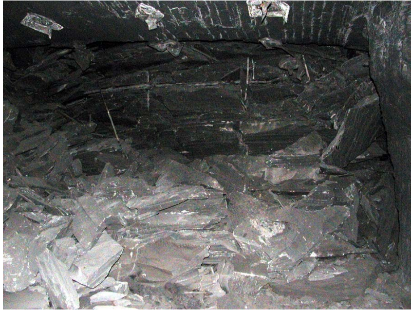
Photo 1. Roof fall in Old 2 nd Left Section. In some cases, a determination of whether the fall occurred before or after the explosion could be made by the relative abundance of soot covering it. A heavy soot typically covered falls that occurred before (or possibly during) the explosion.
