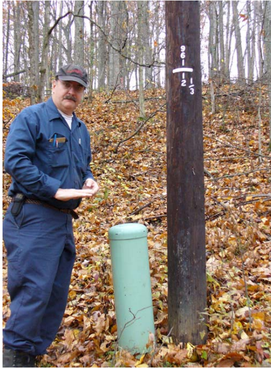
Photo 14: Junction box of 1970's line (closest box to lightning-struck poplar tree.
