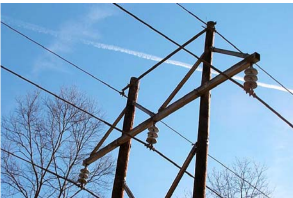
Photo 10. This two pole structure is butt-grounded at each pole. Note “antenna” atop each pole.
