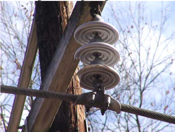
Photo 8. Damaged insulators on the middle phase wire on the main 12KV line
