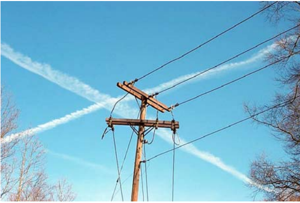
Photo 6. The 12KV branch line is approximately 1 mile in length line feeding the Sago Sub-station.
